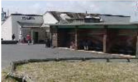
Secluded hidden shelter with little natural surveillance
